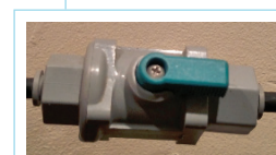
Emergency water shut-off
